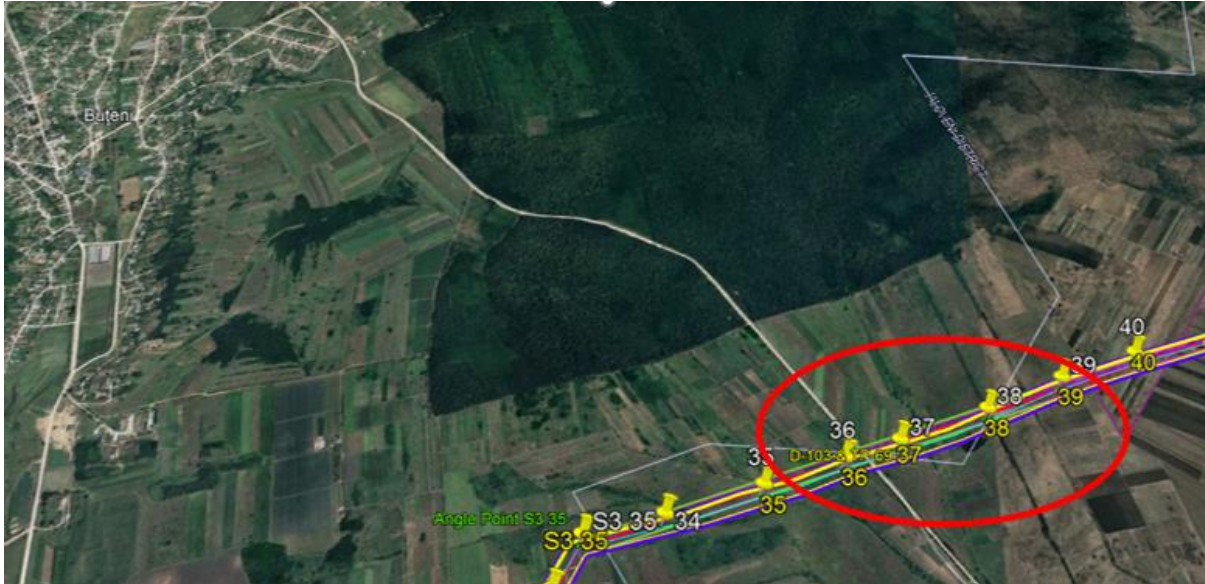
Fig. 3-2: The 400 kV OHTL passes on the territory of the village Buteni, District Hancesti
